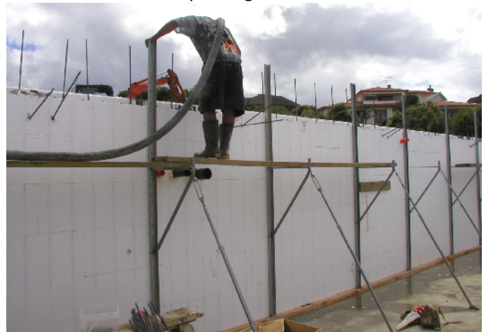
and pouring concrete...
