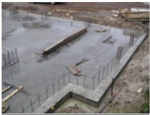
Check on the requirements in your specifications but it would be normal practice to wrap polytene running under the slab to at least ground level on the footing and foundations. Either waterproof behind the polythene using something like 'Sika BlackSeal Plus Bitumen' Waterproofing Membrane or use Autex 3000 that is self-glued to the polystyrene and have it go over the upturned polythene. Penetrations that go through the foundation polystyrene can be surrounded with Wurth Purlogicfor extra seal.
