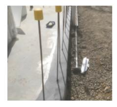
A typical waterproof paint / polythene wrap picture showing it covering all the outside edge of the building. With the new H1 regulations this outside perimeter must now include sufficient insulation to achieve R1.1 See picture of rebated blocks below if the wall construction is in timber.
