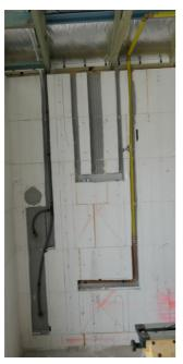
Pipes and wires can be cut into the polystyrene as shown. A hot blade shaped in a loop can form the chaser in the polystyrene. Make sure that the wire is rated for contact with polystyrene. (Usually its purple coated)
