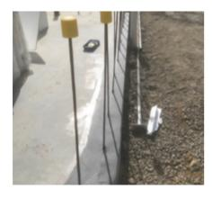
A typical waterproof paint / polythene wrap picture showing it covering all the outside edge of the building. With the new H1 regulations this outside perimeter must now include sufficient insulation to achieve R1.1 See picture of rebated blocks below if the wall construction is in timber.
