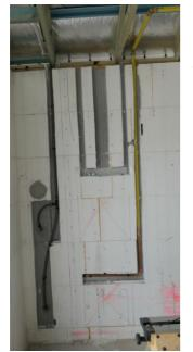
Pipes and wires can be cut into the polystyrene as shown. A hot blade shaped in a loop can form the chaser in the
